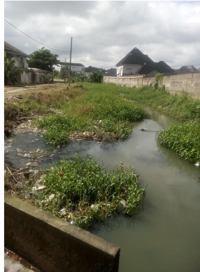
Fig. 3. House structures erected close to drainage channel and weeds taken over the Ntanwogba creek due to indiscriminate discharge of wastes into the drains.
